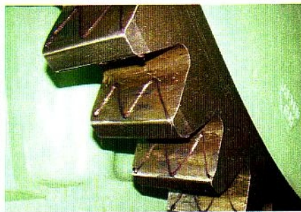
Application of LE 5182 PYROSHIELD on Tooth Flanks of Flywheel
