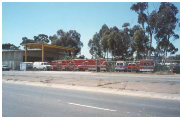
Backside of maintenance facility
