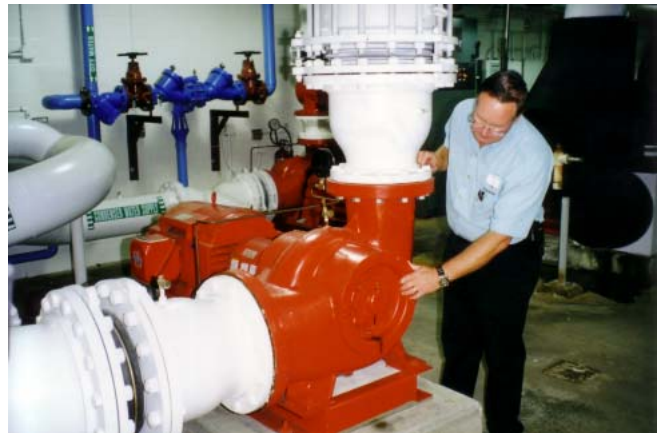
Bell & Gossit pump moves 3,200 gallons of chilled water per minute to the live animal attractions.
