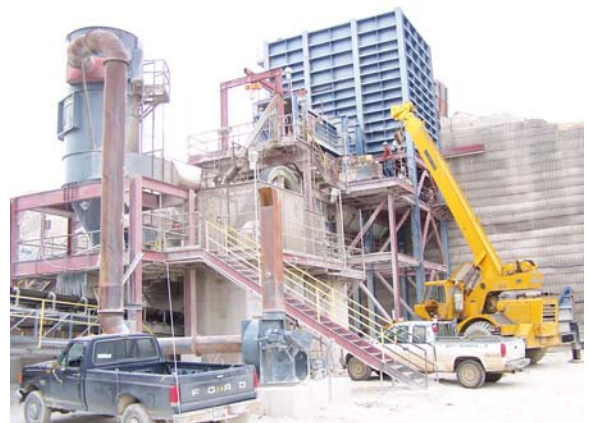
Primary crusher structure
