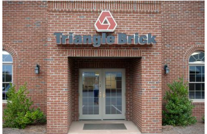
Wadesboro plant office
